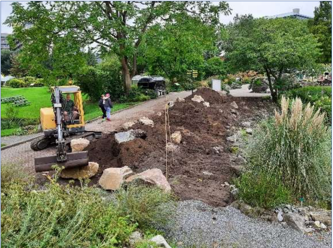
All stones removed and the soil moved into position. Large rocks being placed.
